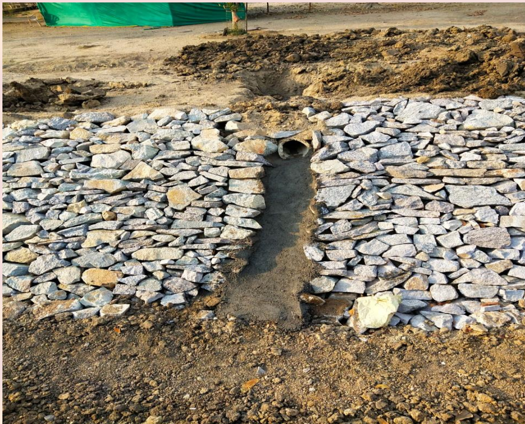
Revetment to the Sambar Deer enclosure Moat
